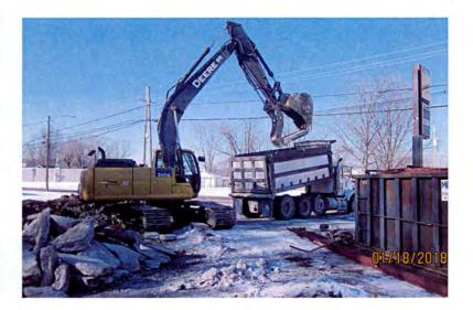
2. Concrete covering the UST tankhold and product piping trench was removed and piled on-site until disposal.
