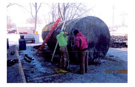
USTs were ventilated with compressed air until the meter testing the lower explosive limit was consistently below 5% under supervision of the Illinois State Fire Marshal representative. Once achieved, USTs were removed from the tankhold and cut before cleaning.
