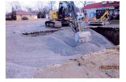
9. After the removal of the USTs and contaminated soils, clean backfill materials were hauled to the site and filled into the tank pit excavation.
