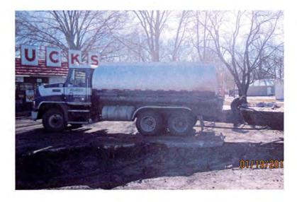
8. Impacted groundwater from the UST tankhold and tank liquids from the site were removed and properly disposed of by First American Recovery and Recycle, Inc
