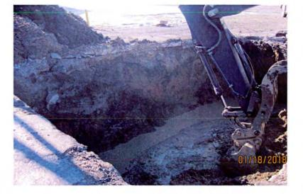
6. Petroleum contaminated soils were hauled and properly disposed of by Charles H. Carter & Son, Inc. at the Wayne County Landfill. Groundwater exhibiting a petroleum sheen was encountered in the UST tankhold.
