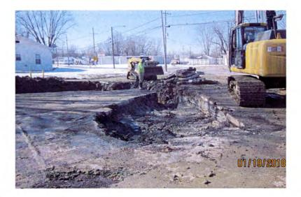
7. The associated product piping and contaminated soils from the piping trench was removed under the supervision of the Illinois State Fire Marshal representative.
