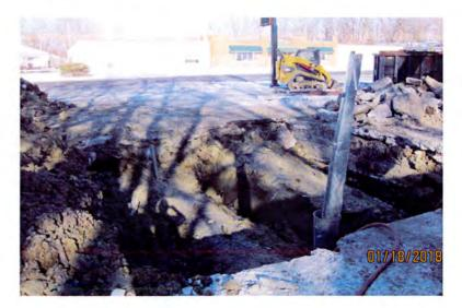
1. The USTs were uncovered and liquids removed. Liquids were pumped from the USTs and associated product piping and stored on-site in 55-gallon drums until properly disposed of by First American Recovery and Recycle, Inc.
